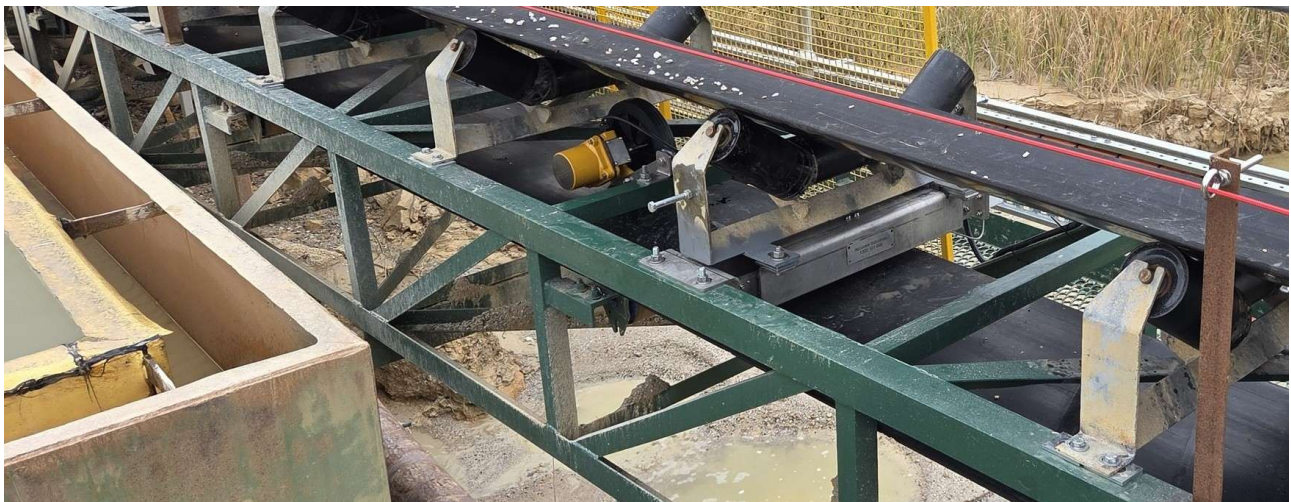
CBW installed on site
